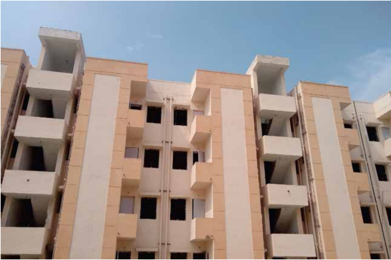
DLF GARDEN CITY LUCKNOW EWS/LIG EXTERNAL VIEW
