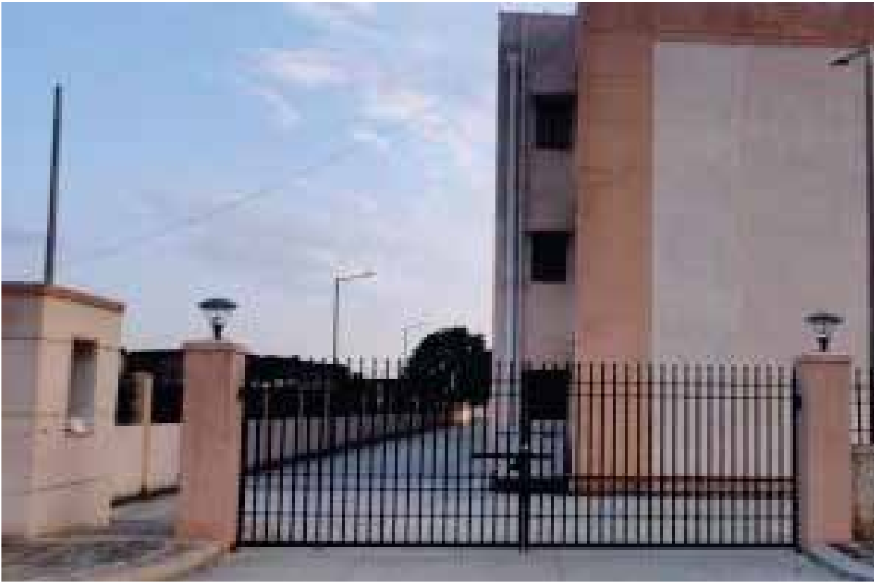
DLF GARDEN CITY LUCKNOW EWS/LIG MAIN GATE & FOOTPATH
